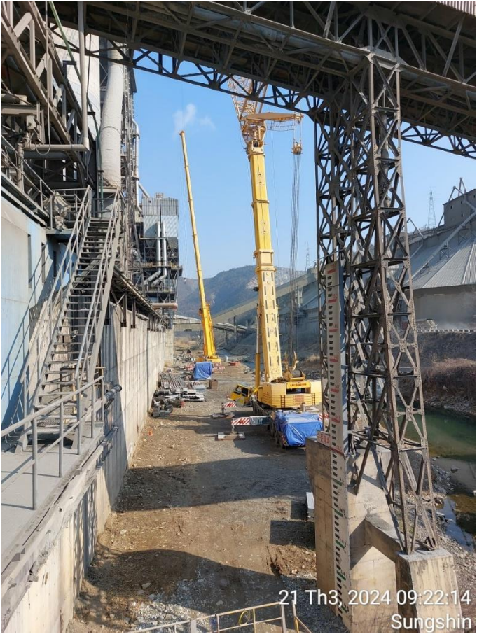
mobile cranes for lifting the equipment
