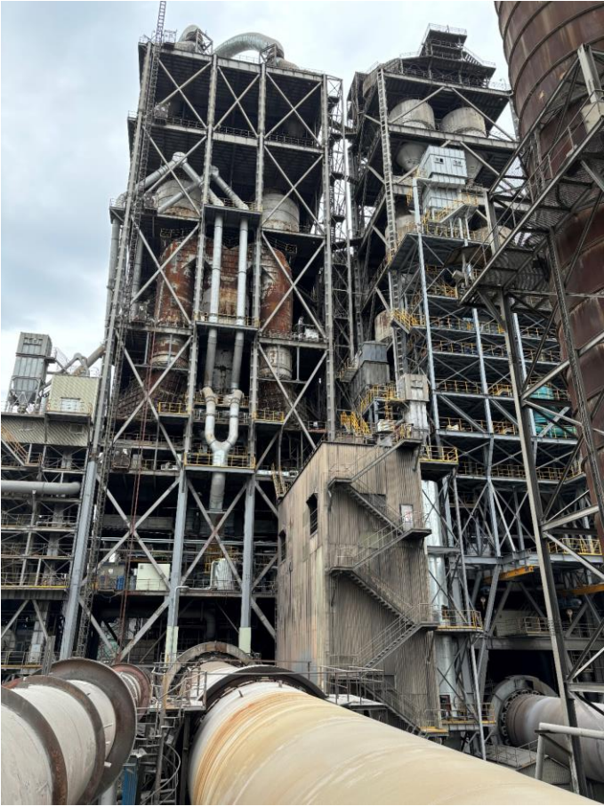
Preheater tower Line no. 5 (left)
